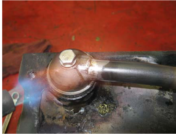
Heat the parts...not the solder
